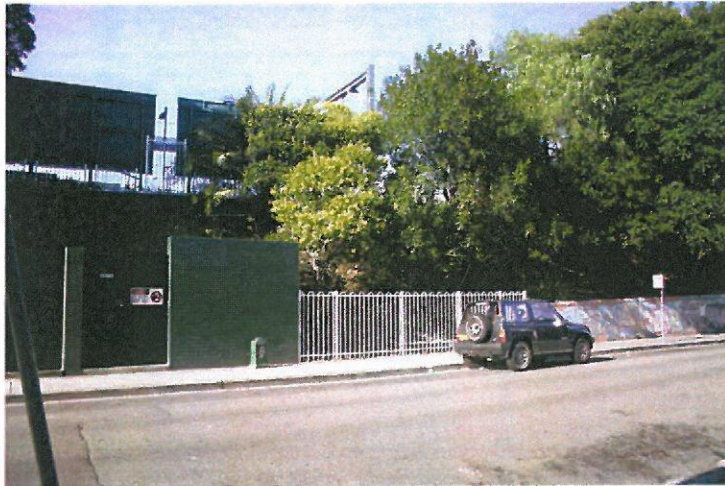
Plate 2 - view of railway corridor showing electricity substation and brick retaining wall
